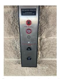
Replaced panel and major electrical / mechanical components to meet fire code:
